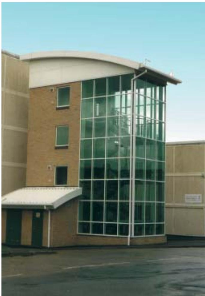
Napier Square is a four storey complex of flats built in 1971, using a concrete panel system, and they were substantially refurbished during the early 1990's.
