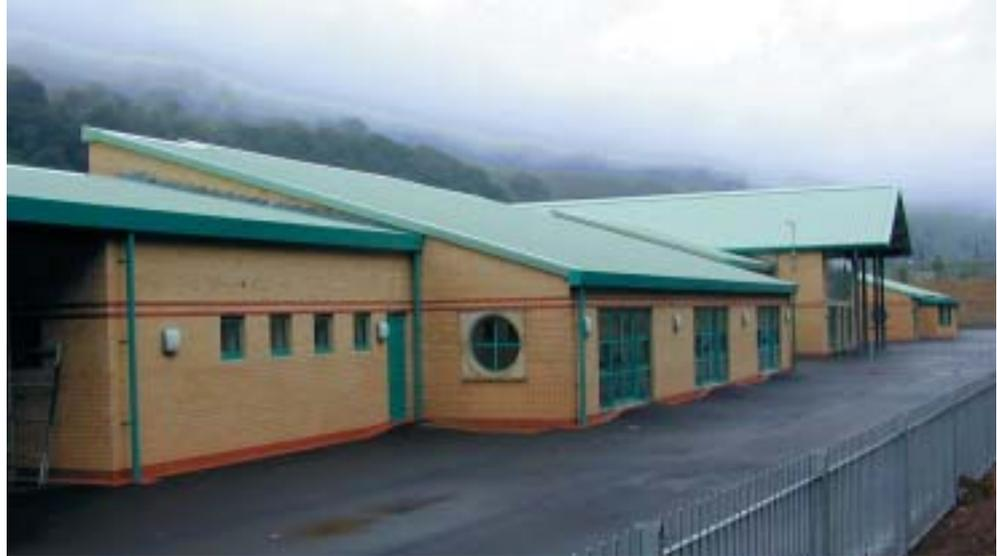
Roof construction comprises a profiled metal deck, supported off a system of decorated glulam timber beams giving a feature of sloping ceilings to the majority of rooms.
