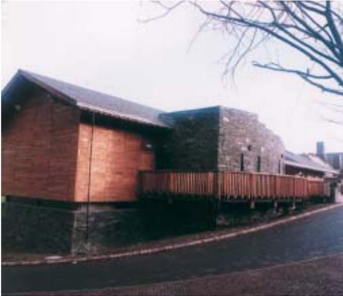
blockwork, and clad externally in a heavy battered stone wall of reclaimed Welsh slate obtained from a local quarry, where it was collected and sorted from the giant waste spoil heaps created over time as a byproduct of the quarrying process. The upper level is a lightweight, 'infill' construction of 200 deep Masonite studs filled with Warmcell (recycled newspaper) insulation and is clad externally with sawn oak boarding. The roof of sawn oak rafters is clad in Welsh Portmadoc slates.
